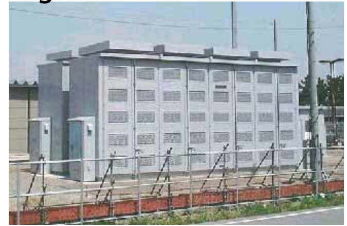
Sodium Sulfur (NAS) Battery
